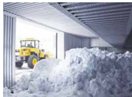
A snow chamber at the Okudaisen Bunanomori Water Plant
