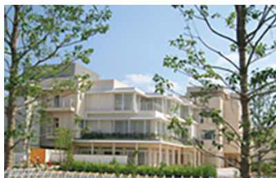
Domyoji-Takadonoen, a general-purpose welfare facility
